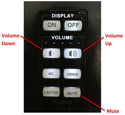
When you are finished, press the OFF button to shut down the room.
