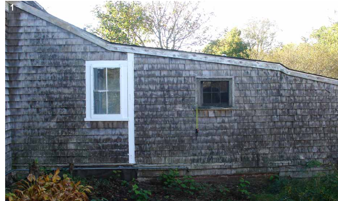
1. The exterior ell on the western elevation was constructed at three different times.
