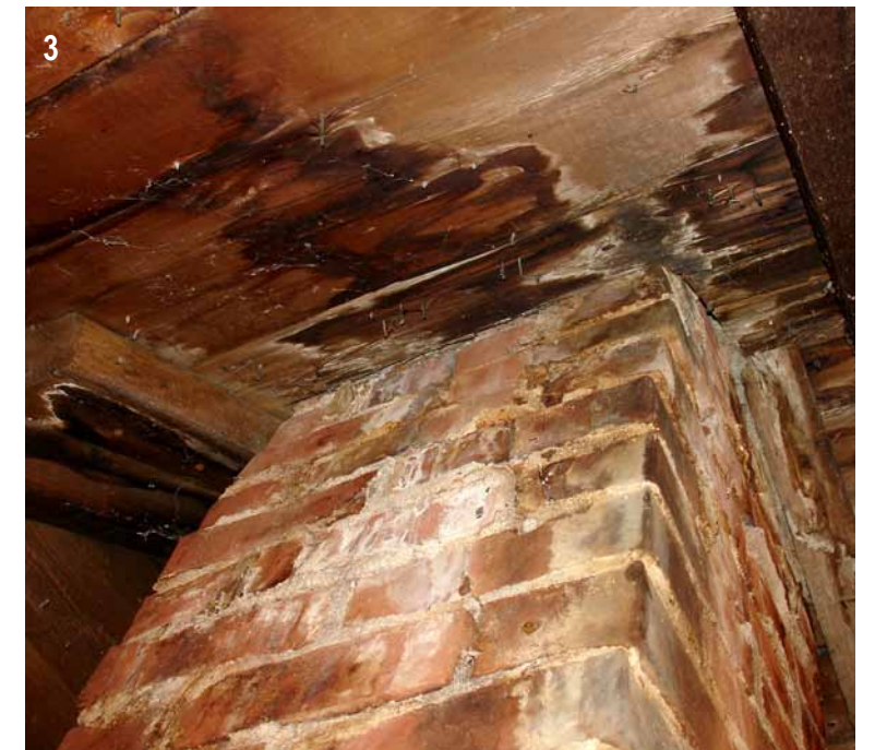
3. Chimney in northern ell shows signs of cracking and moisture damage.
