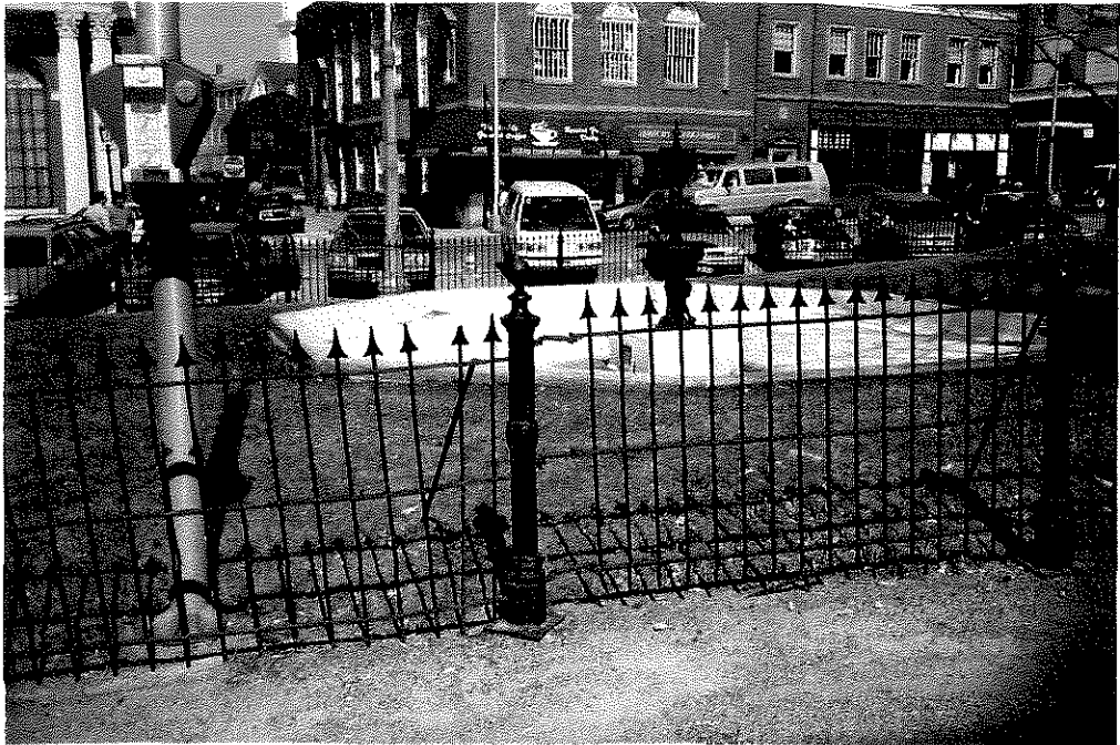
Embedded posts and lower rails; poor quality rail restoration
