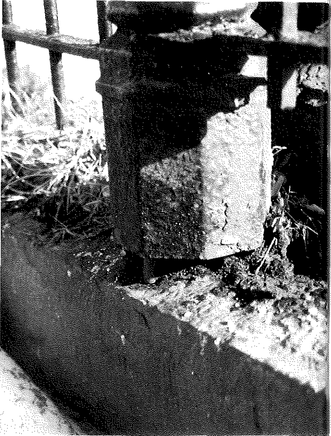
Original mount system in poor condition
