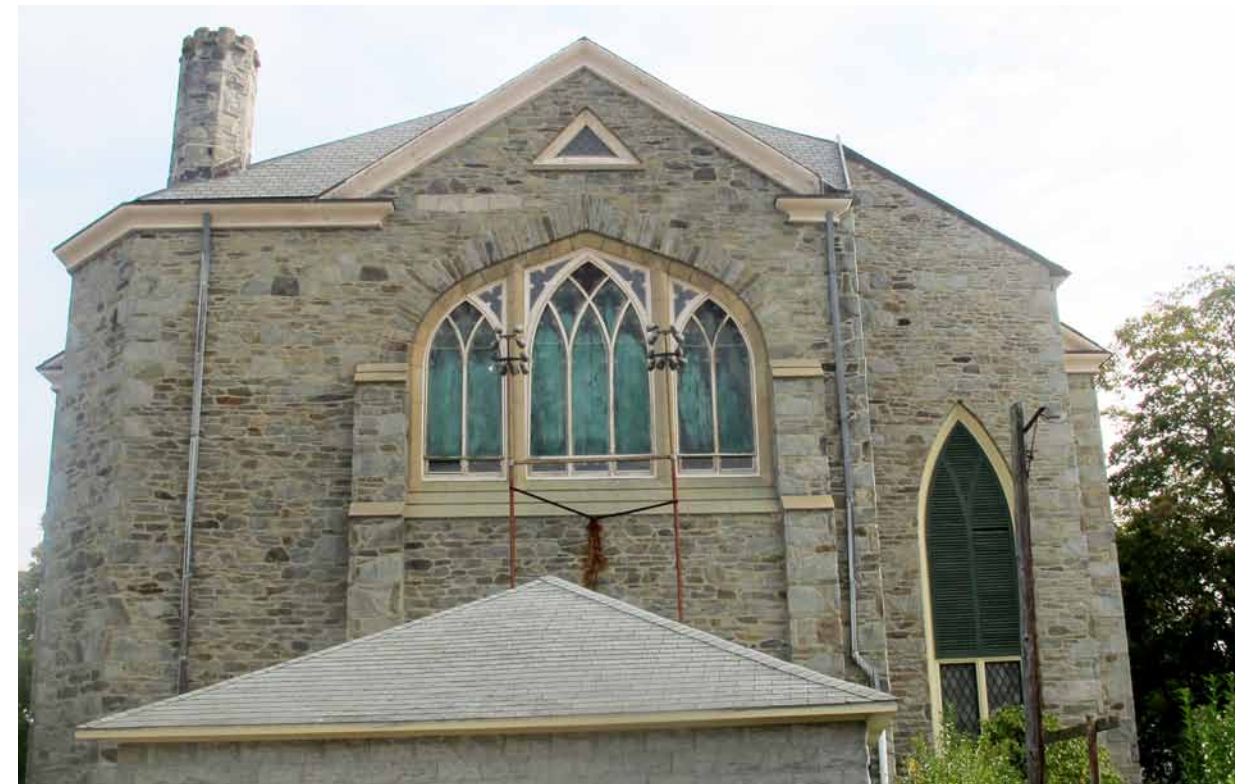
West elevation shows some stone wall rust staining, which needs to be cleaned.
