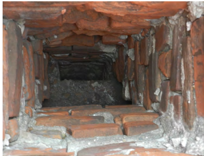
Advanced deterioration of interior of east chimney.
