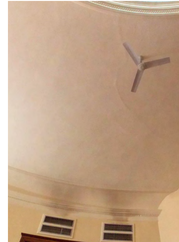
Ceiling paint failure and staining from vents to be analyzed and addressed.
