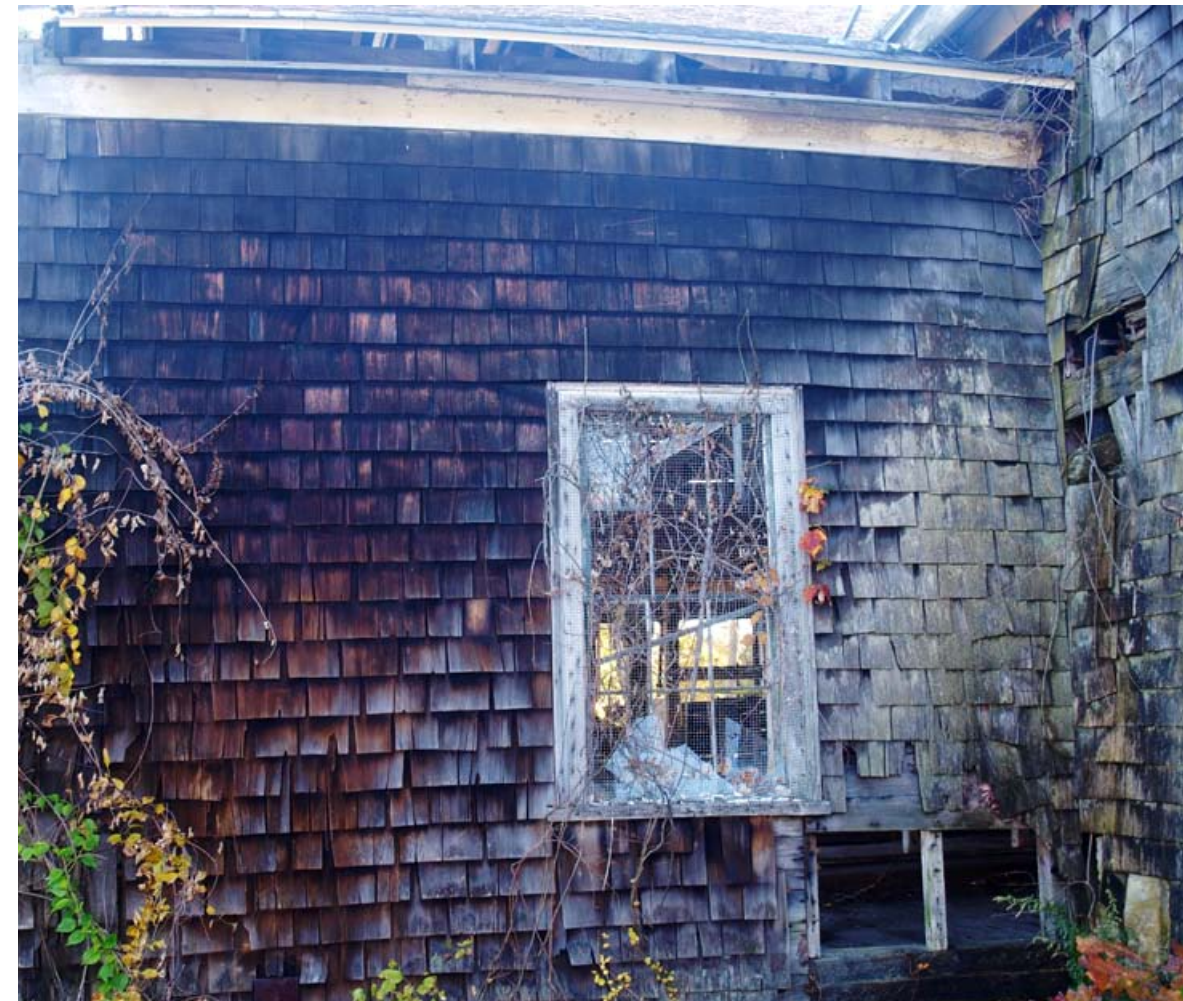
The south and west elevations of the barn will be entirely re-shingled with true cedar shingles to exactly match the historical finish.
