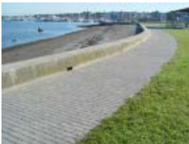
Newly paved walk in King Park
