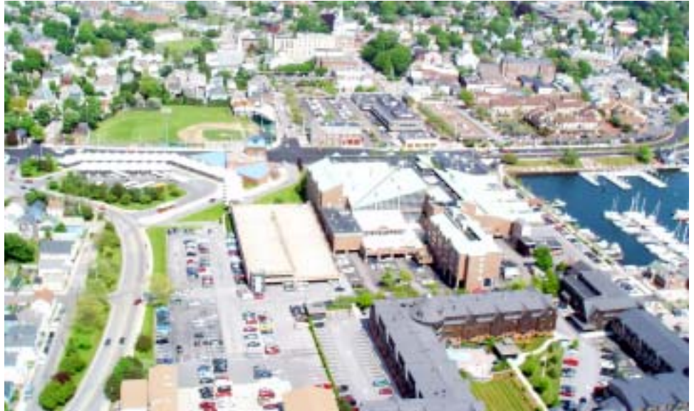
Aerial view of Gateway Center
