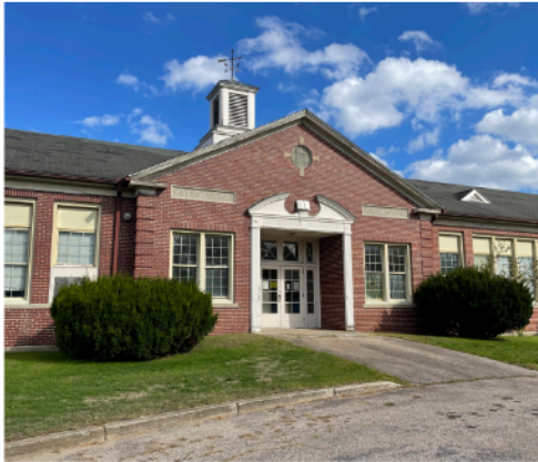
Former James Oldham Elementary School, 640 Bullocks Point Boulevard, East Providence
